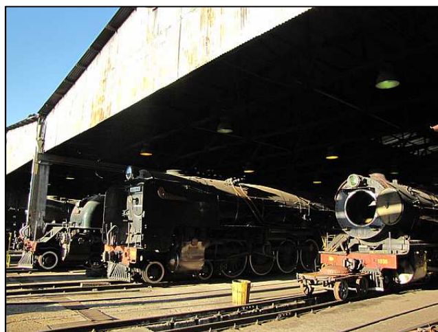
P215 - The Germiston Steam Depot was originally founded circa 1895. Nearly 120 years later and a changed country later, the core of the old steam depot has survived as a functioning concern. It is truly a remarkable achievement!
