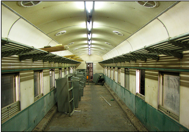
P03 - Although weathered from exposure, and still a bit caked with limestone from her days at a cement plant, the interior isn't in bad shape. It has been stripped to allow better access for a THIRD cleaning, a repaint in our two-town brown scheme and to have new floor coverings laid.
