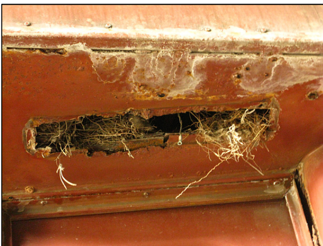
P11 - Union Carriage and Wagon duplex accommodation. Bird's nests in one of the vestibule light apertures. The entire roof of the coach is coated with baked-on lime dust from the Cimpor Cement Factory which stored this coach. This coach will likely need abrasive or chemical treatment to clean the roof for a proper well-bonded re-paint.
