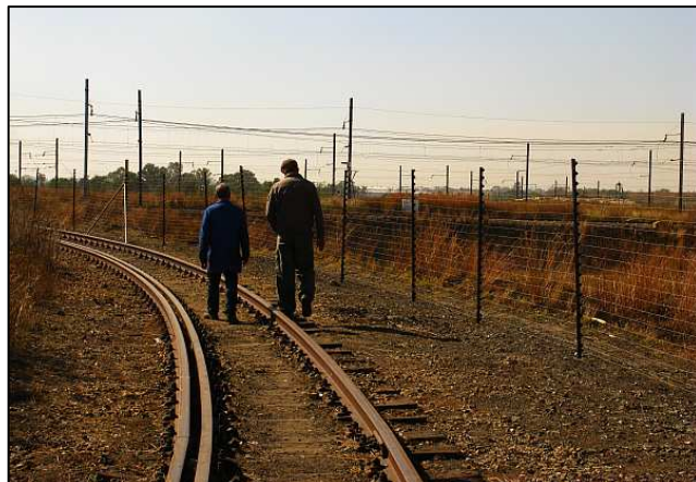
P02 - Gordon and Shaun are discussing the coming repairs to the turning balloon. The sleepers are rotten in several places, the track has a few kinks and many of the fittings and bolts for the check rail (inner rail) have been stolen.
