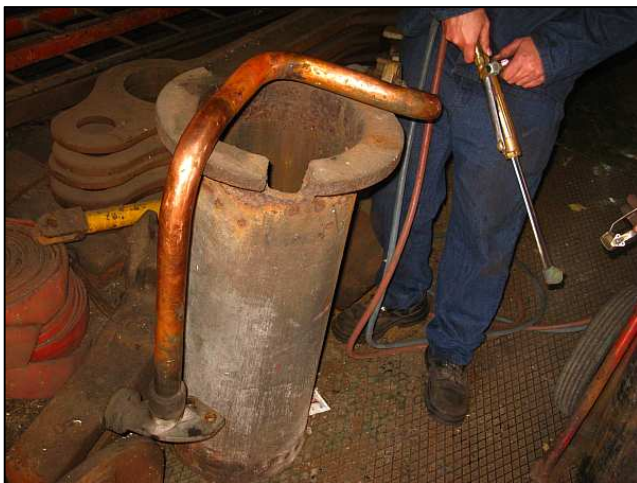
P27 - Another view of the riser pipe being set up for annealing. Big bore copper pipe bending and fitting an inevitable task in steam locomotive restoration, even when transferring parts and pipes between supposedly identical locomotives or from stock.
