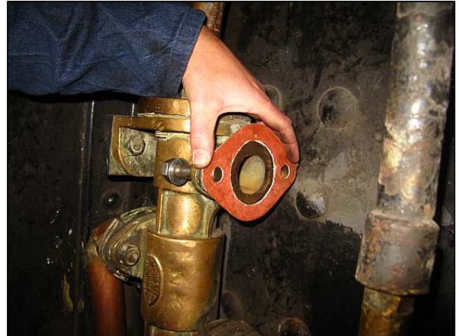
P14 - Oops! The flange measurements were taken from the flange of the copper riser pipe and one would naturally assume that the holes are the same. (They DO match on the fireman's side) The bore of the injector's water inlet is significantly smaller even though the flange bolts match up.
