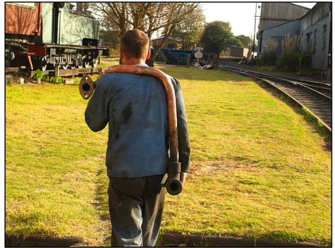
P26 - The need to keep the flanges and bolt holes parallel and to extend the swan neck meant many trips to the 'annealing shop' in the Millsite Store. The lovely Jeandrette demonstrates the fashionable copper pipe boa.
