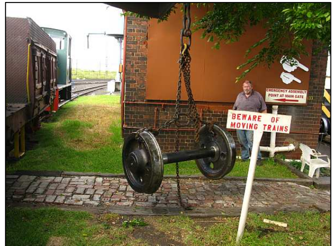
P16 - Beware of moving axles. The end of the first drag becomes a hovering swing to avoid the sign before setting the axle down again. The slings and the lower chains needed to be removed to shorten the chains for the final lift.
