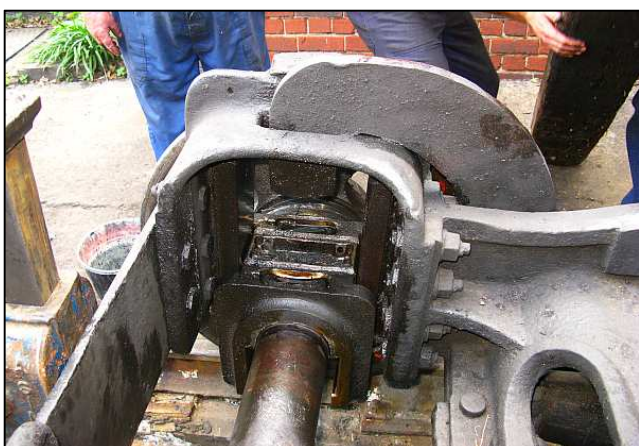
P11 - As soon as the tips of the equalizer beam clear its recess, the brass oil lids were removed from the oil basins set within the crown of the bearing.
