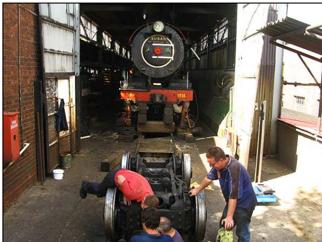
P01 - With the front bogie rolled out and the wheels safely chocked ('Scotched') it was now time to start jacking the bogie up to get the axle horns clear of the front axle bearings. We could have used a wheel pit to just 'drop' the axle, but wanted to expose the whole bogie for servicing.
