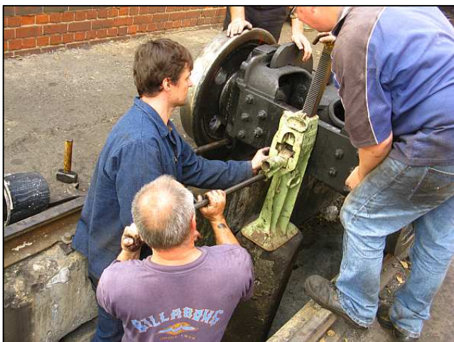
P07 - The bolt came out reluctantly but then jammed when its threads met the frame. The keep and its 'core' bolt was tilting upwards slightly. A click-clack jack was brought out to lift the frame relative to that keep and to use the weight of the axle (still on the rail) to press the keep down slightly. It worked and the bolt was then withdrawn by hand.
