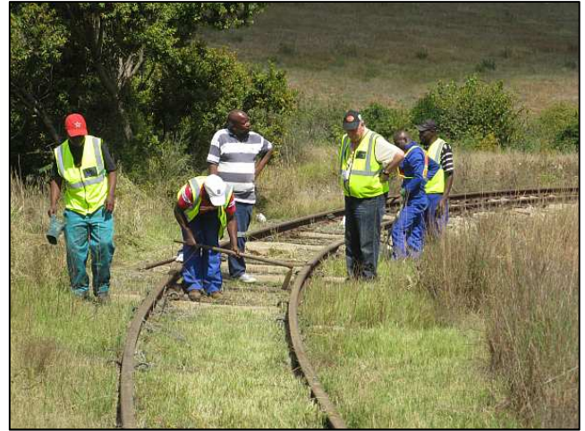
P08 - Joe's team didn't have so much growth to deal with at trackside, but the track itself was overgrown. Grass in the ballast hinders the drainage and dislodges the stones.
