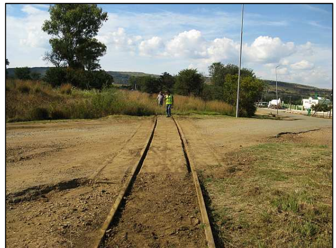
P12 - One of the two road crossings with newly cleaned-out flangeways. Now let's see if our drivers can keep the anvils on the rails instead of the roads!
