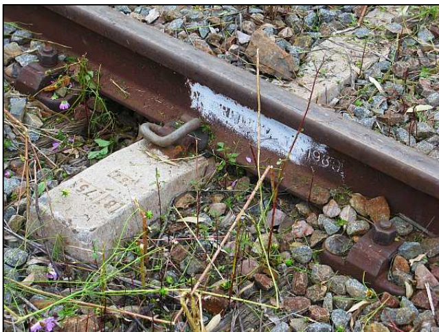
P15 - This rail was rolled in 1939 and likely saw service on the old Pretoria main. By contrast, the concrete sleeper was cast in 1975. Note the hodgepodge of Pandrol clip (left) and rail clamps. (right) Transnet will still replace the wooden sleepers for us in the event of their failure or theft.
