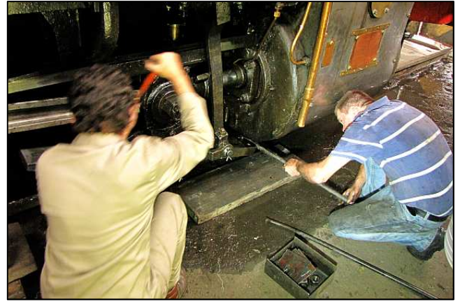
P08 - Even with the rear cylinder cock removed, the bar was still snagged-up. The problem was that the crosshead wasn't forward enough – although going too far forward would get the horizontal union link mixed up into the works.
