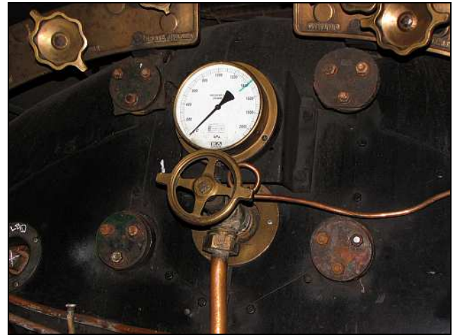
W10 – A bit bare on the backhead.
