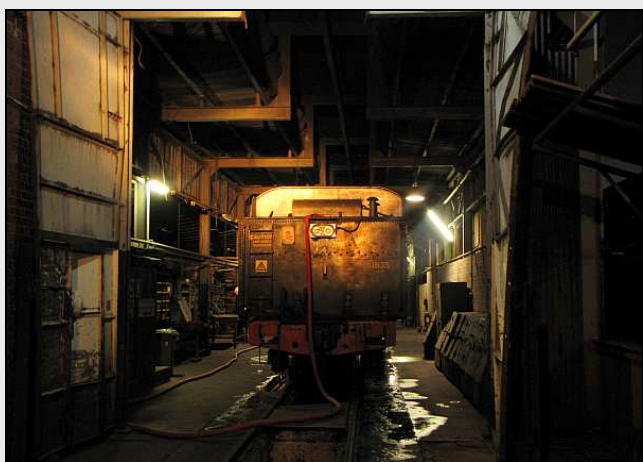
P21 – With three big anvils in residence, the loco minders had a scramble to find hoses to trickle charge their tenders. This hose topping off the 12AR’s tender is coupled to one of a pair of droppers that are actually gravity-fed from the water tower just outside, rather than from the water mains.
