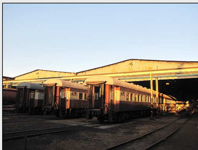
P28 – The 15M workshop looked distinctly odd with three bays just stuffed full of coaches. We had to have two tracks clear up at the top end. The opportunity was taken to get the rest of the Silver Class Sleeper Coaches down here for their upgrades for the November Steam Tour.
