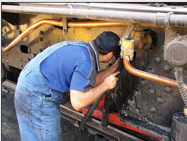
P45 – On the 12AR No.1535, even the roughly painted frame plates had been cleaned and they were reflecting the yellow of the blow down box. Passed Fireman Andre van Dyk is seen washing down the ash pan.
