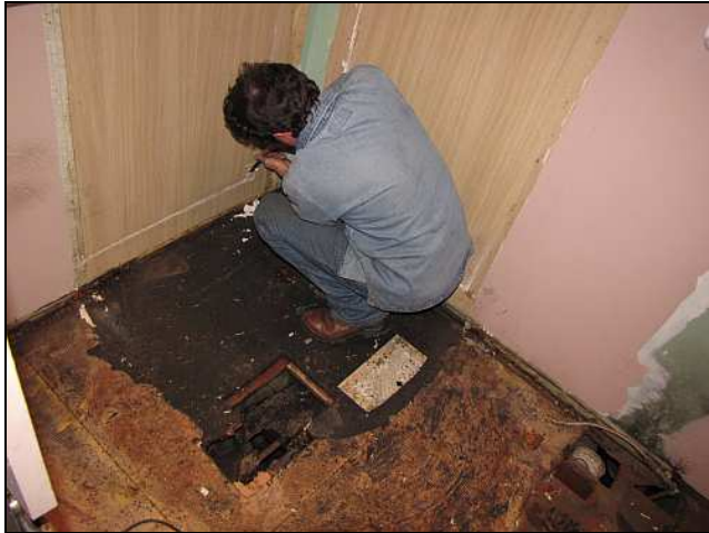
S07 – In Comp C bathroom, Alan scrapes away the stingy single strip of silicone beading from the laminated backing. This floor is in poor state with many extra holes. The triangular-ended hole in the corner is original – it used to be for the Coupe’s compartment’s sink
