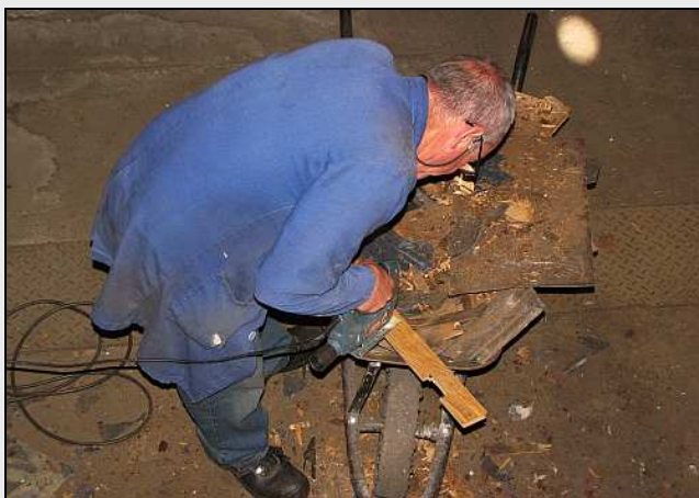
S05 – Gordon uses a barrow to brace both ends of the floor plank that he is trimming for a sink. These prefab T&G planks are labelled as 'laminated,' but they are closer to a 'veneer' with a solid wooden core and laminated coatings.
