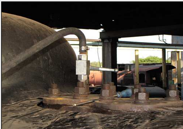
P13 – Even with the piddly blow down spacers leaking on both sides, it was judged worthwhile to pressurize the boiler again. But first, the dodgy venting valve was removed and replaced with this high pressure model. The blanking plates are where the dual safety valves would normally go.
