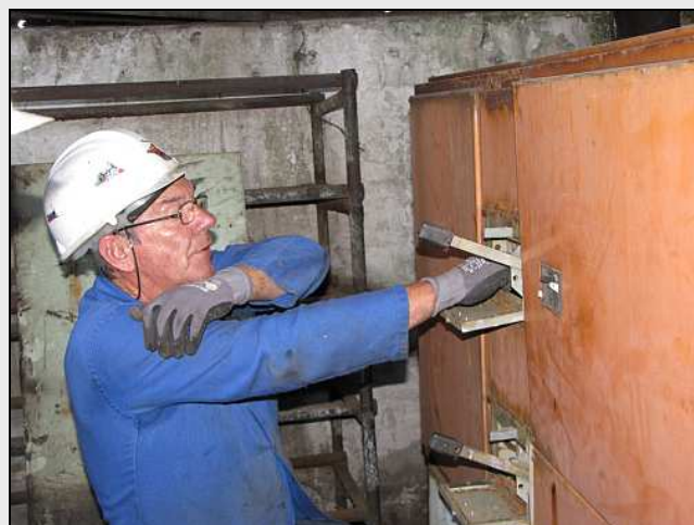
P16 – The wiring for the WAP machine was in bad shape and also had a phase switched with a neutral. It turned out that this board is overfused, and instead of tripping, it allowed the wiring to overheat. Gordon condemned the wiring immediately. Here he is nervously trying to open the fused isolator on the MCC panel in the wheel lathe house. He is deliberately wearing the rubber gloves in this picture.
