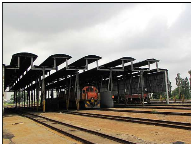
P24 – The future of the Bethlehem Depot is clouded with ever-reducing rail traffic and there may come a day where this place becomes disused and derelict as well. There are only two diesels on shed today and we never saw more than 5 at a time for the entire stay.
