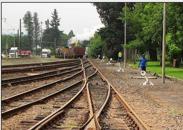
P15 – Looking down the classic single points ladder for the diesel locomotive shed. This backing-up move was to get the coal handling wagon cut off away on its own track for easier access for later if needed. The two diverging tracks in the foreground are for the repair shed and you will notice they are rusty from disuse.
