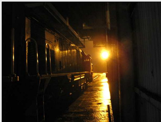
P56 – Clearstory engine sheds are great for letting out coal smoke (and diesel fumes), but they do tend to let in the rain. The trio of diesels and the bays were just as wet as they would have been if they were exposed outside.
