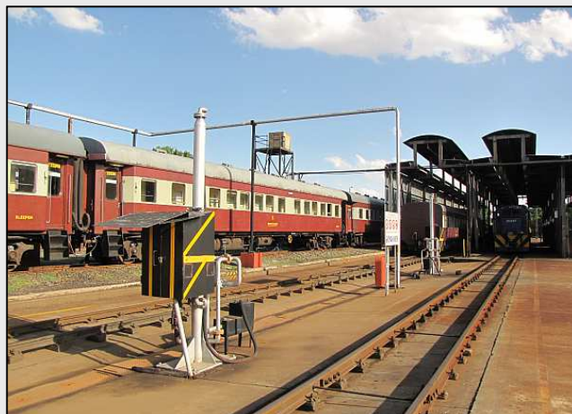
P38 – This was an interesting area to explore ... a still used dual-bowser diesel refuelling station. Only mad men and English dogs would dare to be out in the heat.
